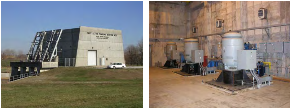
Figure 4.1a & 4.1b: East Alton Number 1 Pump Station
