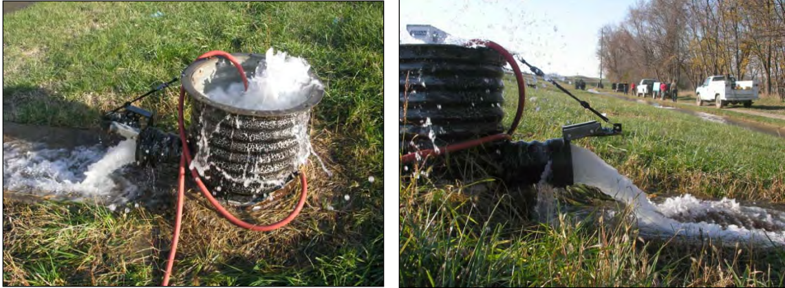
Figures 2.16a and 2.16b – Typical Well Flow During Air Lift Pumping
