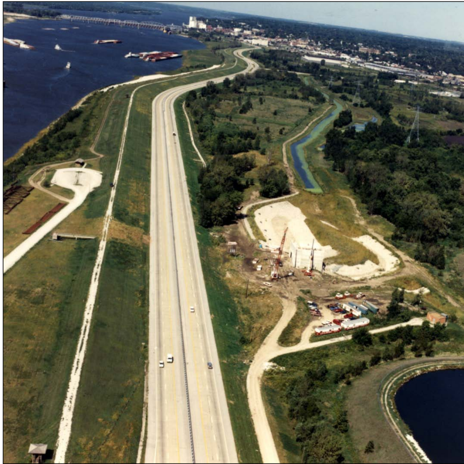
Figure 2.3 – Landside of Wood River Levee (Sept 1988)
