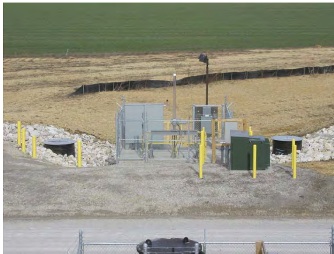
Figure 4.4: Grassy Lake Pump Station
