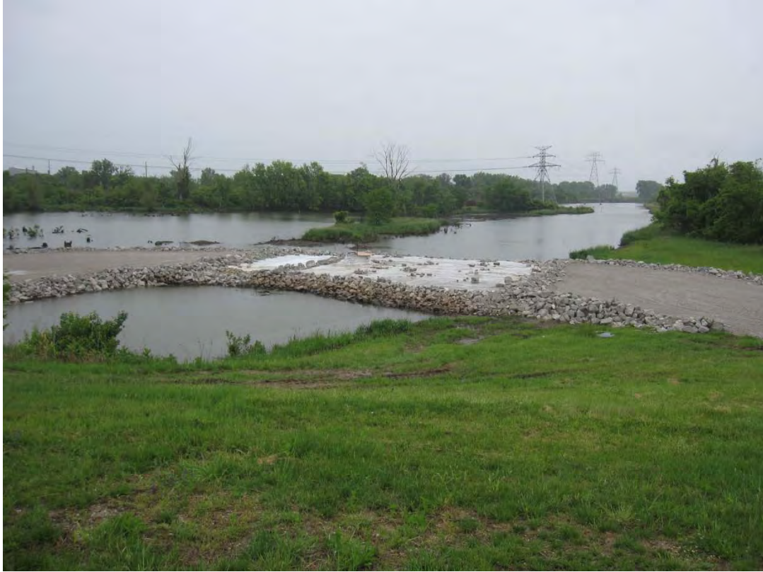
Figure 2.11 – Partially constructed Dike C
