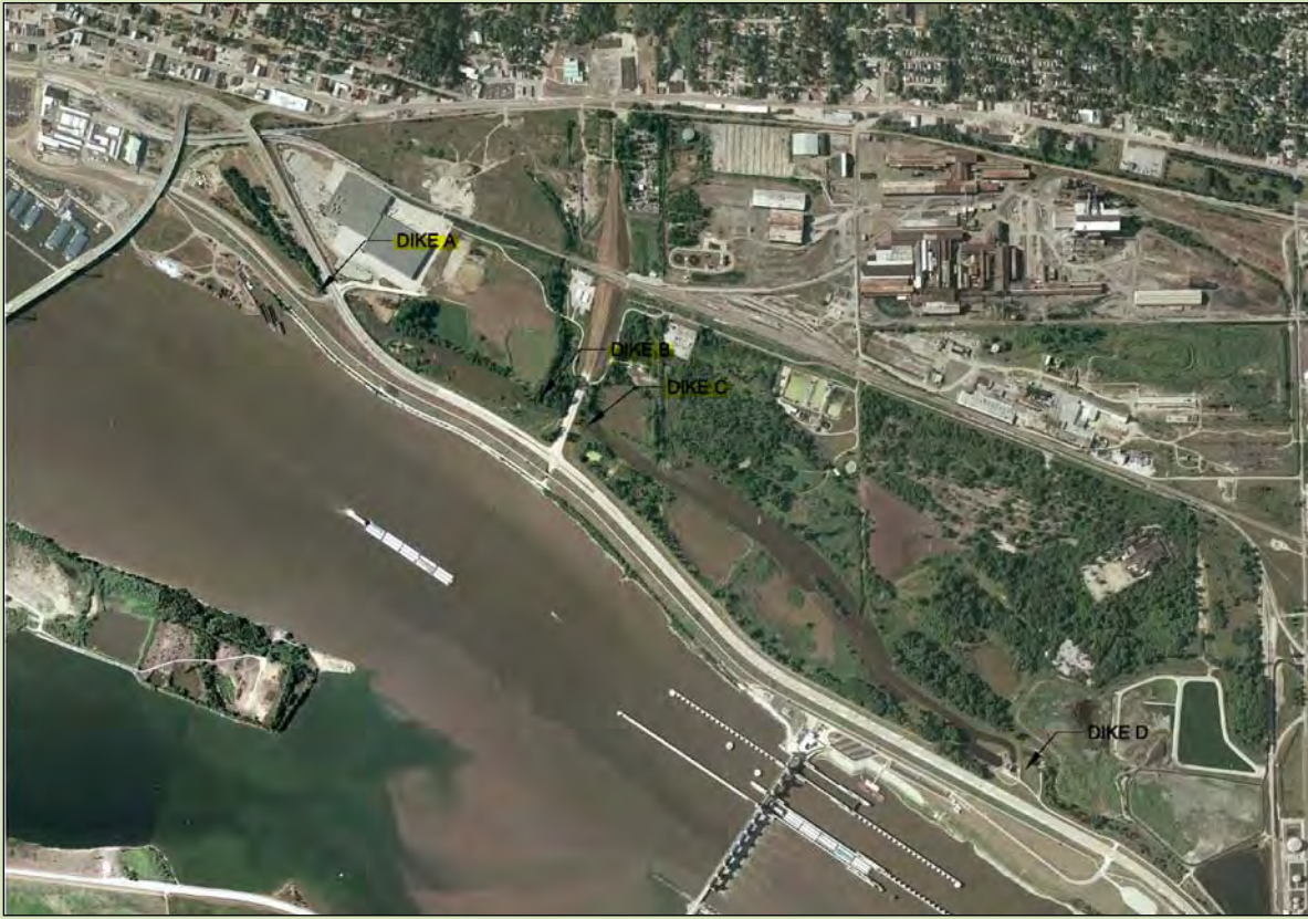
Figure EA-5. Interim Risk Reduction Measures – Location of Three Rock Dikes.
