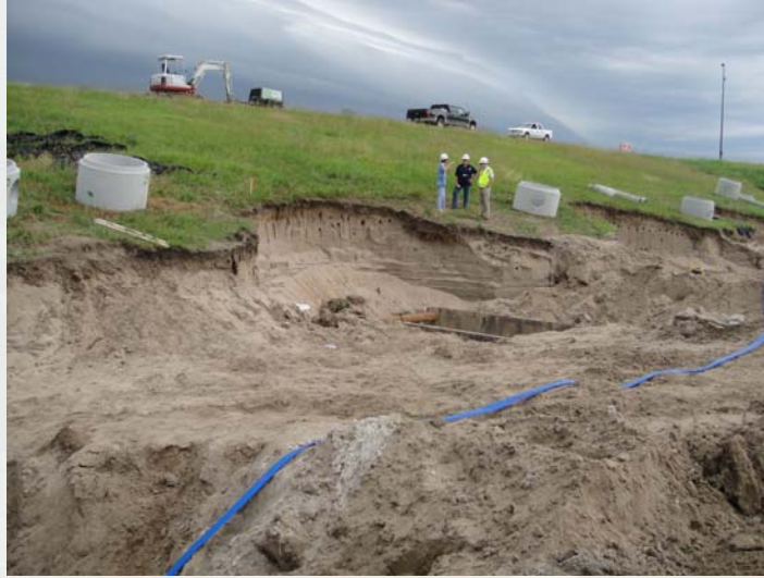
COR south berm underseepage correction.
