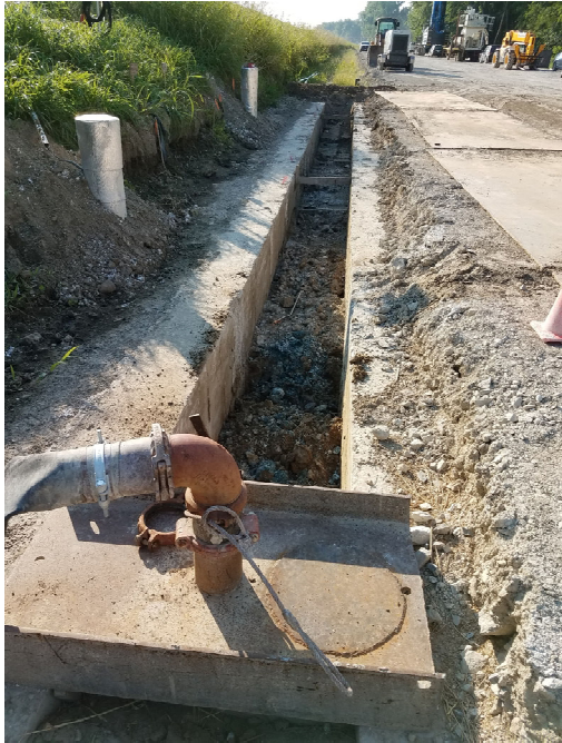
Guide wall installation
