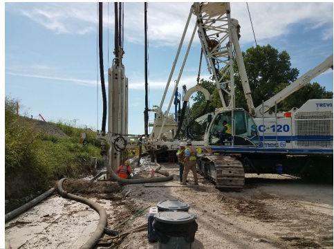
Hydromill Excavation
