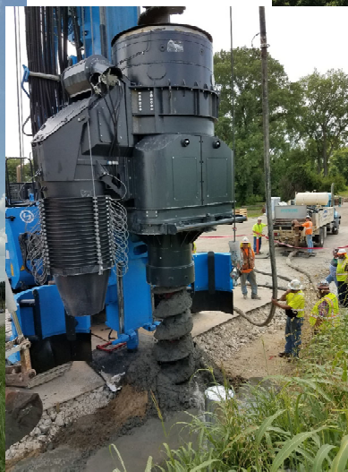
Drilling Cement-Bentonite Columns
