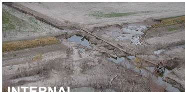
INTERNAL EROSION ALONG OR INTO CULVERTS
