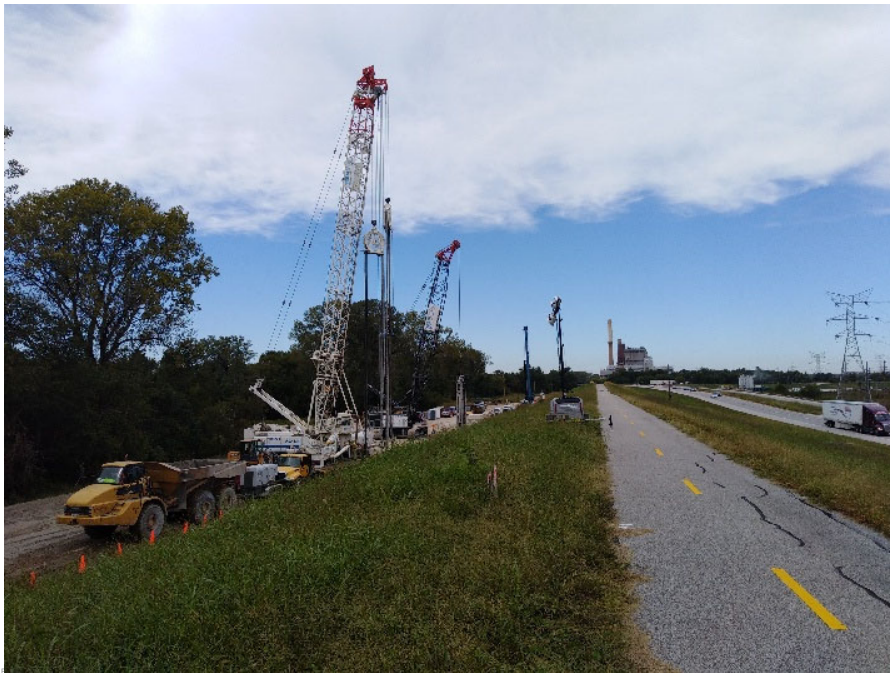
Wood River Deep Cutoff Wall Construction
