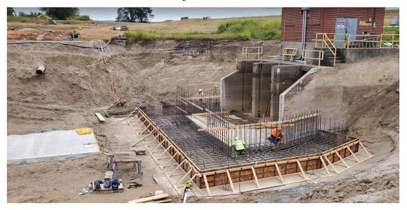
BP18: Placement of First Box Culvert Section
