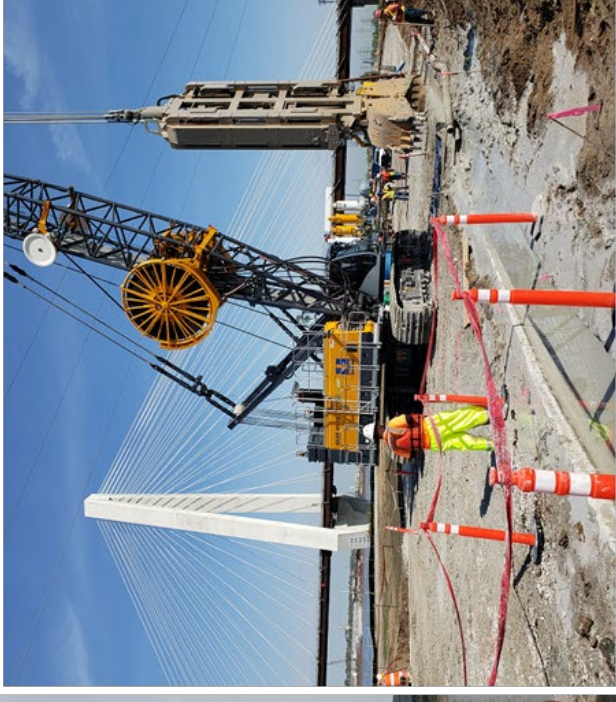
Deep Cutoff Wall Construction
